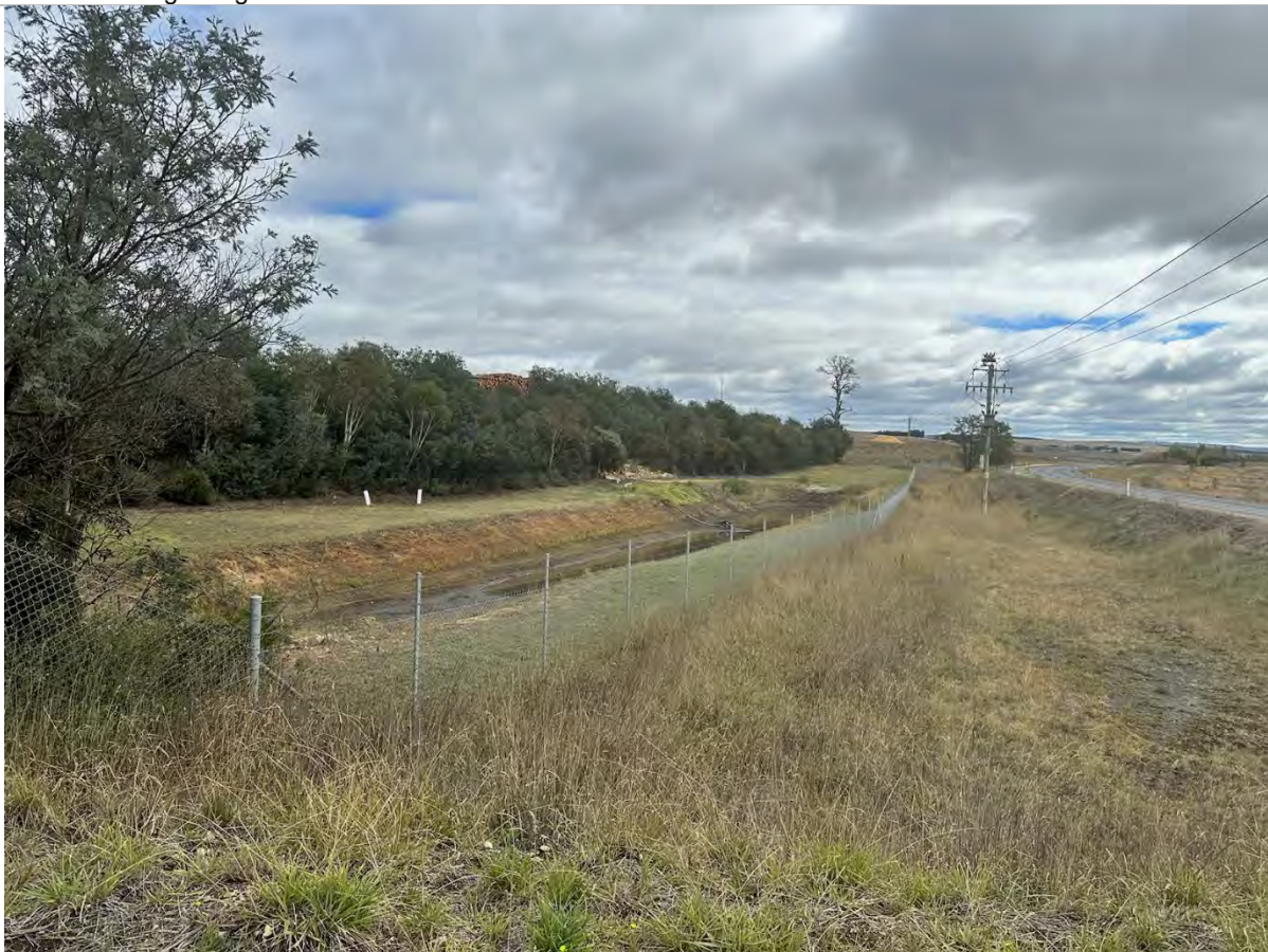
Photo 19: Surface water detention pond
