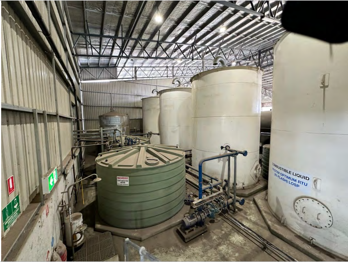
Photo 12: Chemical Storage and bunded area
