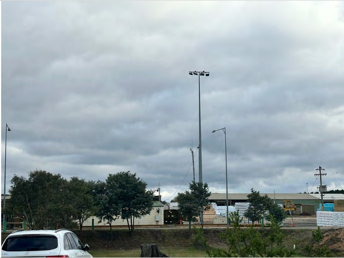
Photo 20: Security and carpark lighting
