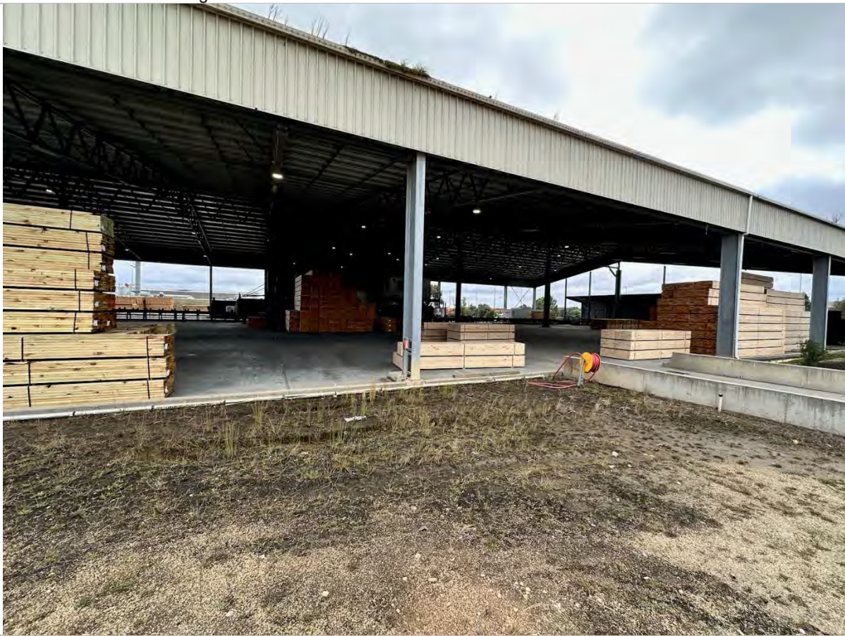
Photo 17: Covered and banded timber treatment and drying area
