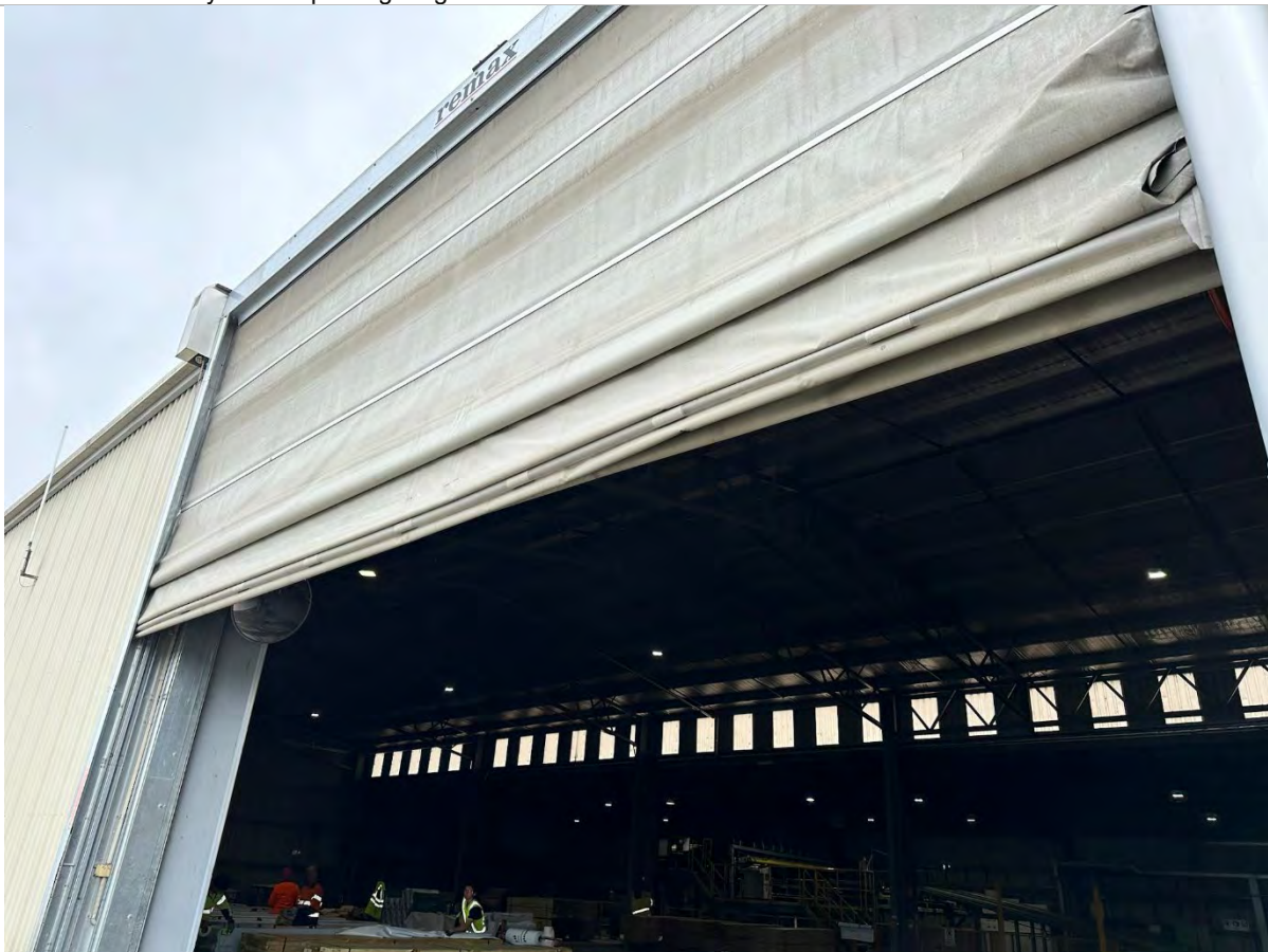
Photo 21: Acoustic roller door
