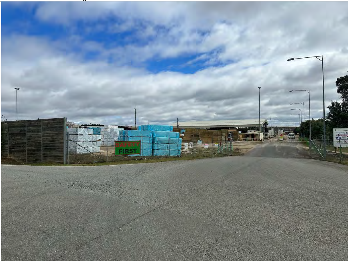
Photo 13: Site exit point with no mud tracking
