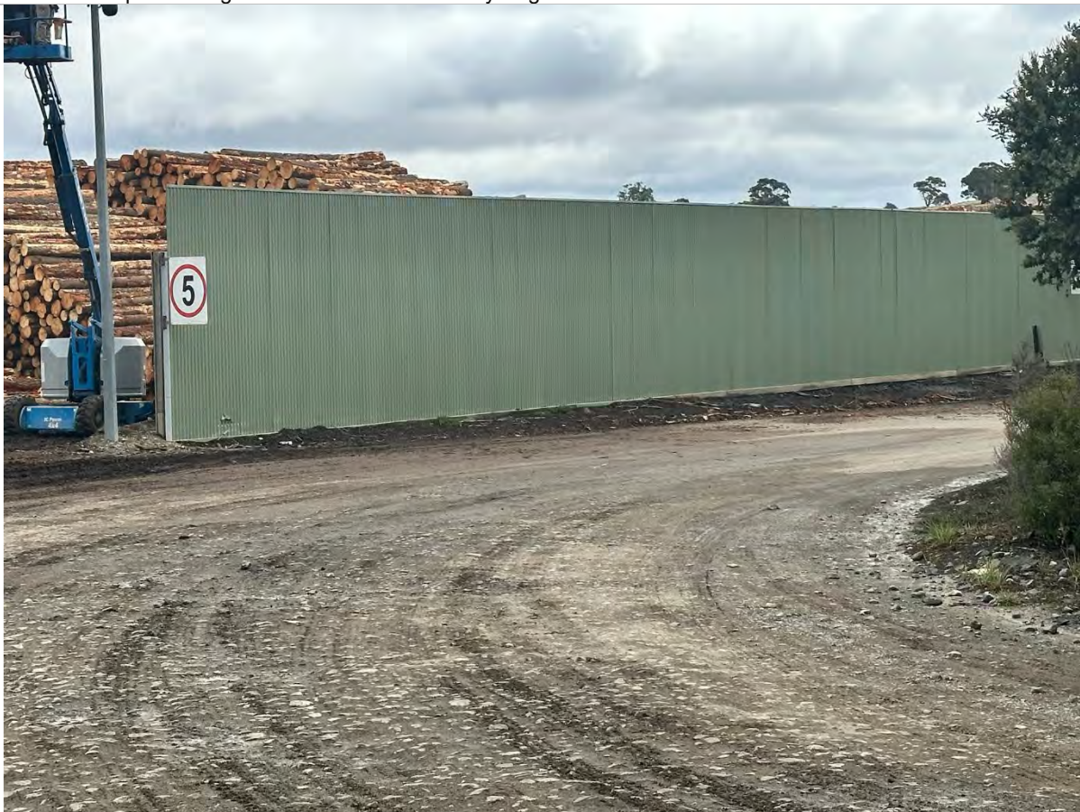
Photo 2: Acoustic hoarding and speed restriction signage
